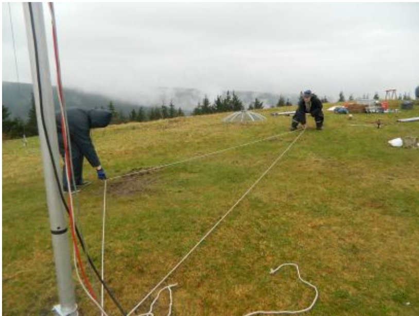
„Egyptian triangular method“ to determine the place of the masts carrying the parabolas. The mast carrying the 23 cm antenna you can see in the front.
